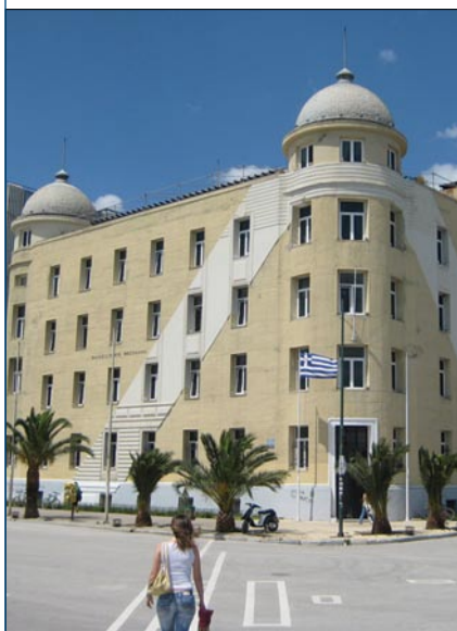
The University of Thessaly (administration building) Volos, Greece.
